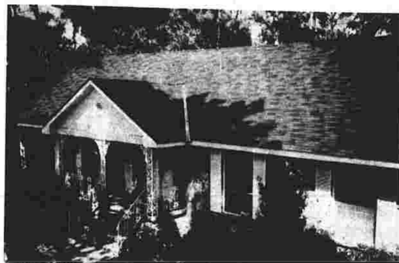
ASPHALT SHINGLES are 36 inches wide with either two cut-outs to create a 3-tab design, or one cut-out to produce a twin-tab design. The GAF Suburban shingles which appear on this roof provide a long, sweeping look and emphasize the width of the house.
